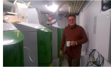
Peter Guenther, Yamori Inn in Norman Wells, NWT showing the new pellet heating system
